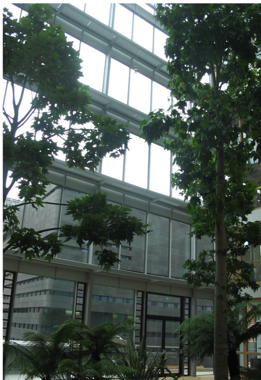
Figure 2 Green Appearance of the eastern atrium
